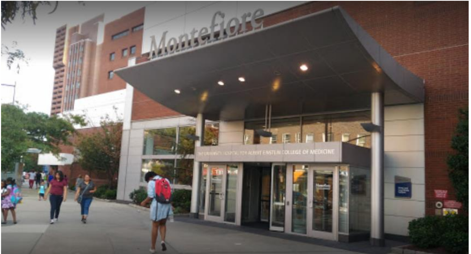
The Children's Hospital at Montefiore, Bronx New York, USA.
